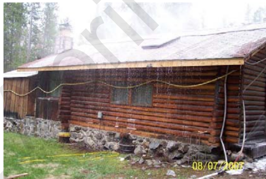
Figure 4-33. Figure 4.13.5B Water Curtain on a Structure During the Pattengail Fire on August 7, 2007.
