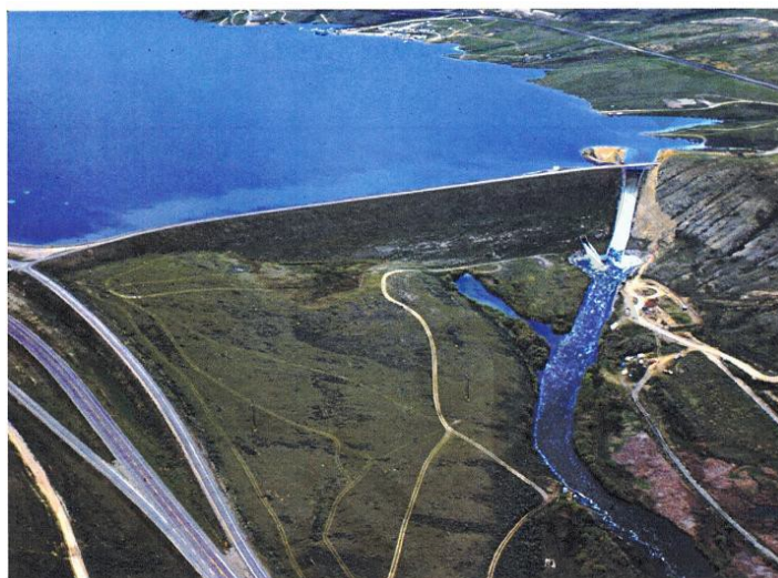
Figure 4-16. Figure 4.5.1E Clark Canyon Dam.
