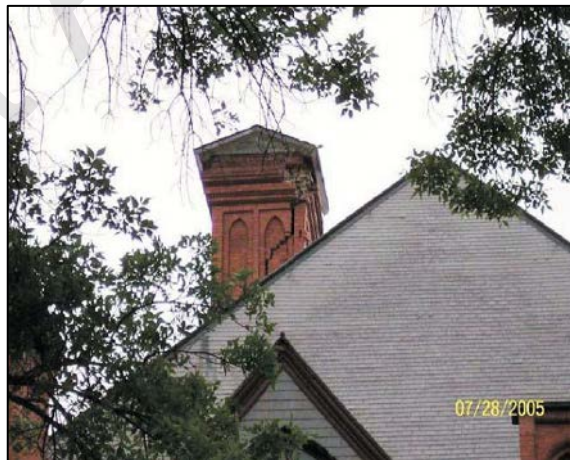
Figure 4-8. Figure 4.4.2A Damaged Chimney of Old Main Hall Following the 2005 Earthquake. The chimney was removed to prevent total collapse. Source: Stickney, no date.
